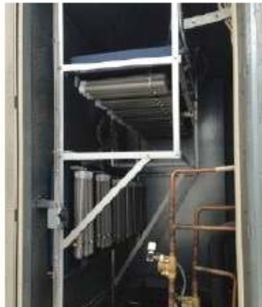
Rack Mounted AHU Supply Plenum
