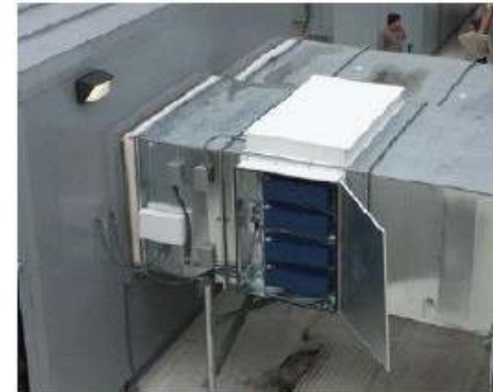
Exterior Duct Mounted with Custom Enclosure
